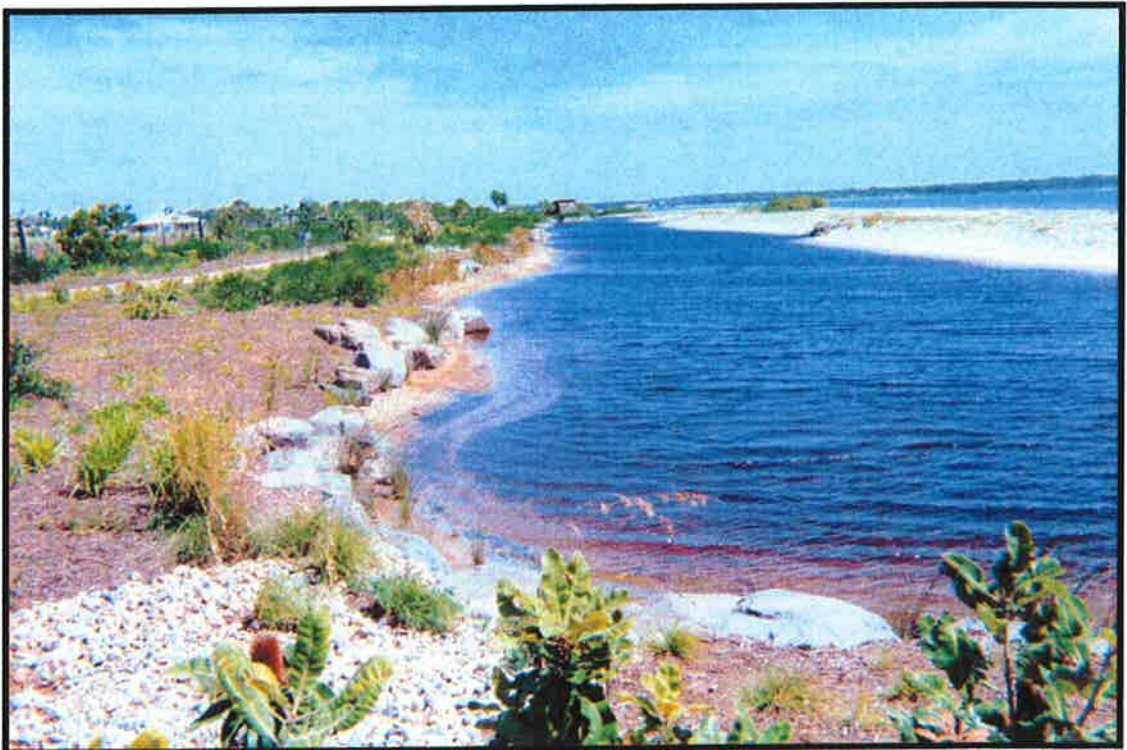
Plate 5b. Use of rocks as erosion control in selected areas around the lagoon margin. View looking south along the lagoon.
