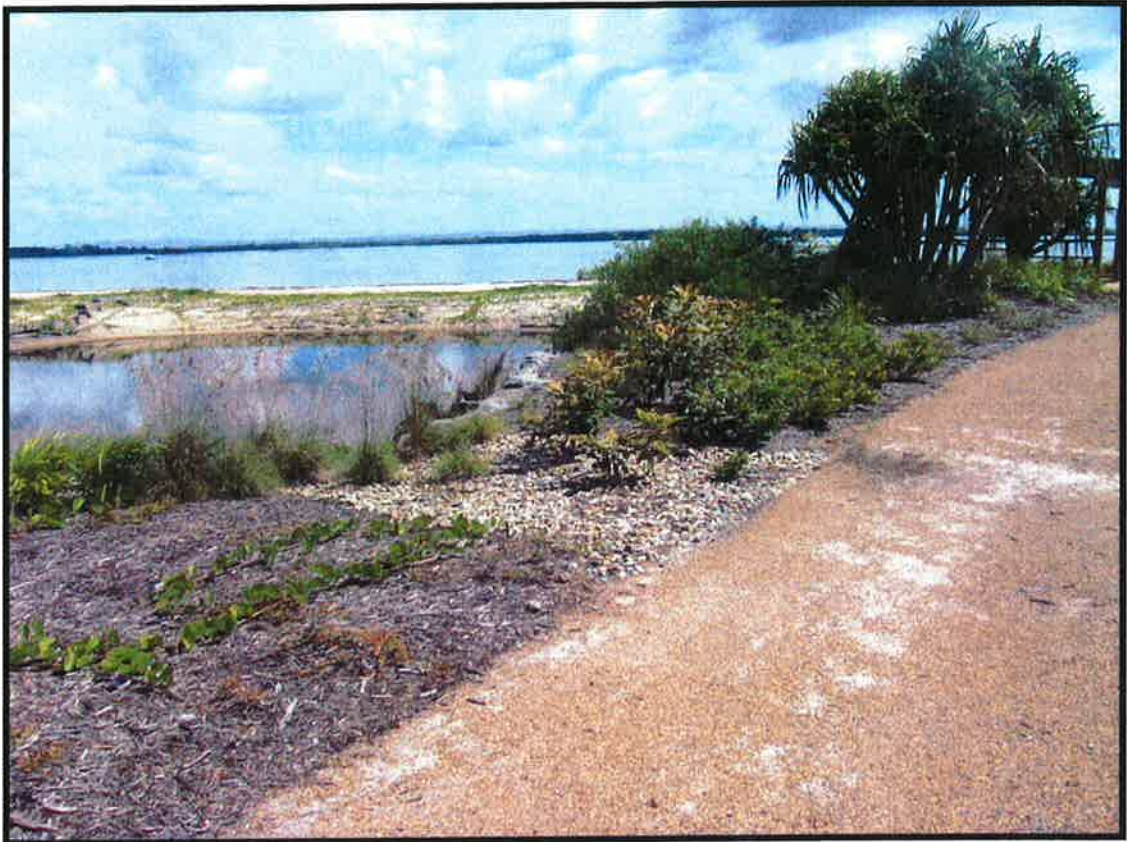
Plate 5a. Use of rocks in the garden bed to dissipate the energy of runoff water in selected areas of the site. Northern end of lagoon.
