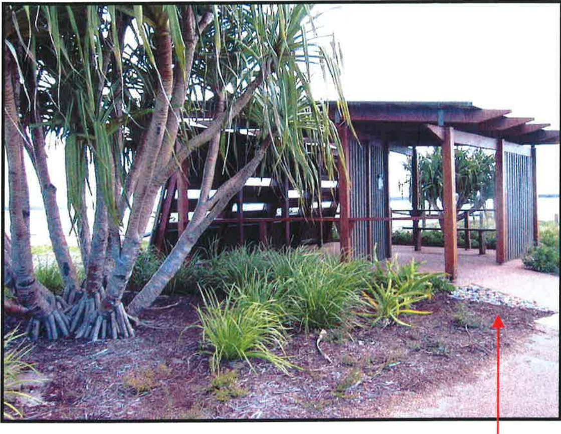
Plate 16. Rocks at base of gutter overflow to minimise erosion from runoff. Bird hide at northern end of site.
