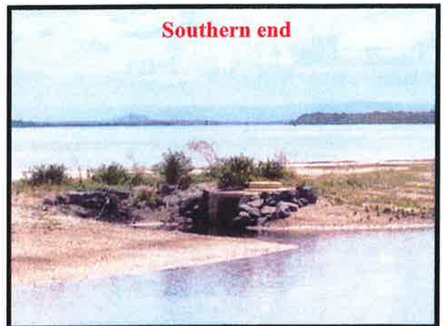
Plate 7. Inlet / outlet weirs on the western bank of the lagoon.
